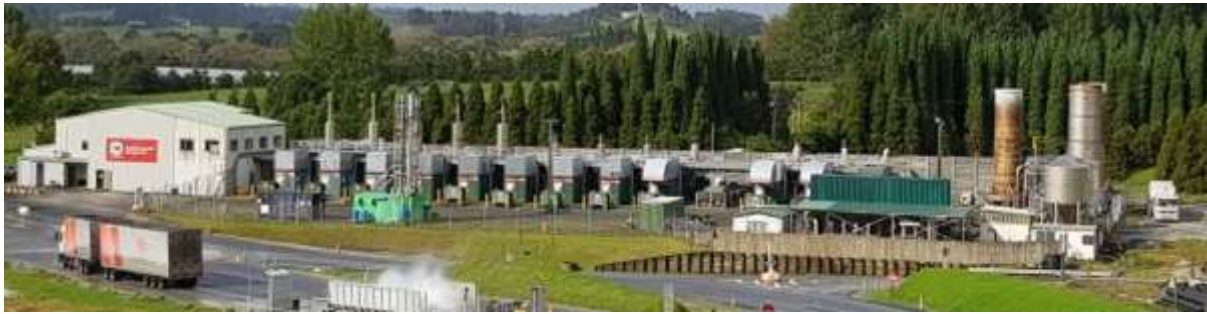
Figure 5.1: Example energy centre, Redvale Landfill
